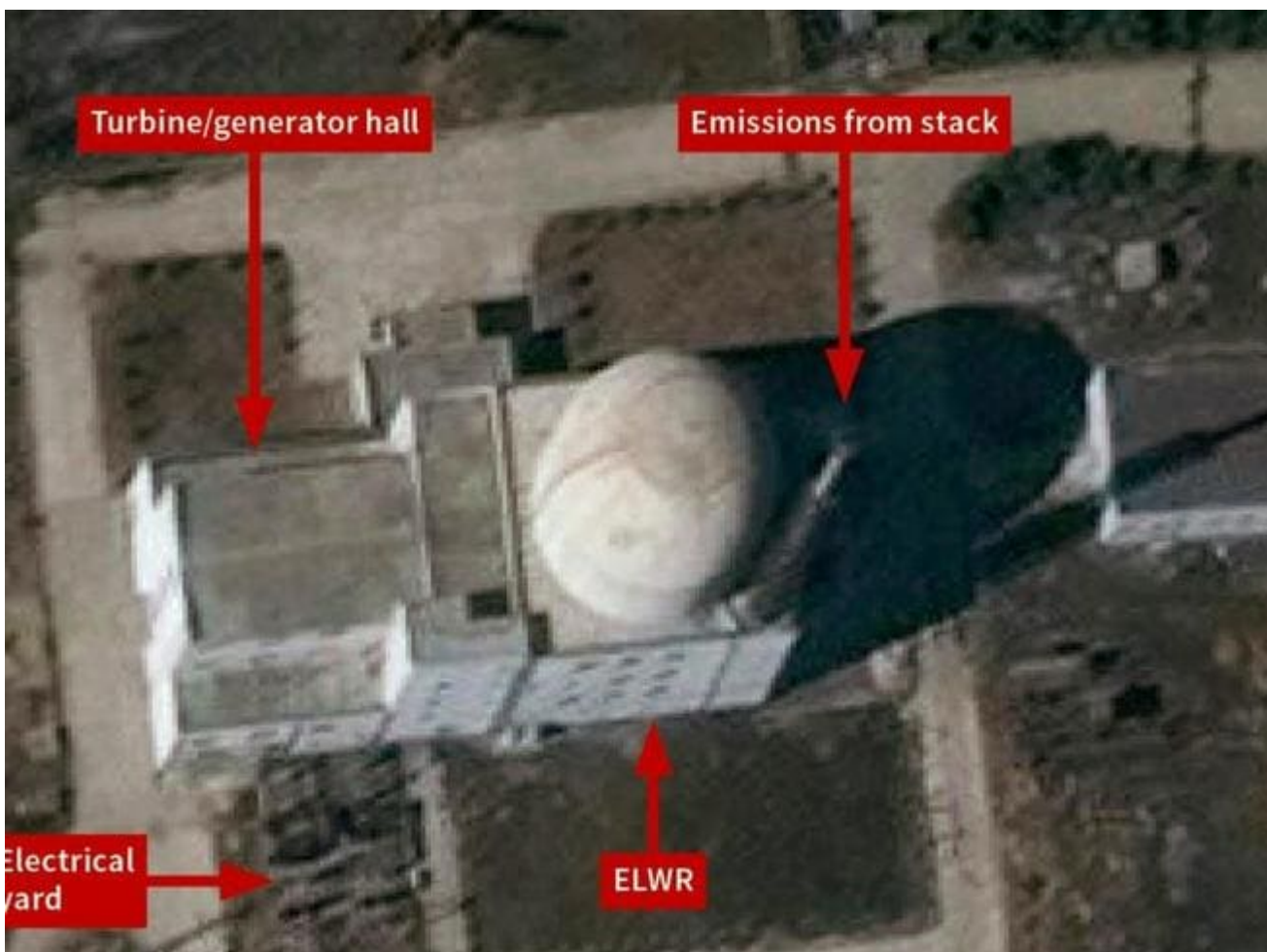
The Yongbyon experimental light water reactor in North Korea, suggesting trial operations are under way. Picture: Associated PressSource:Supplied
