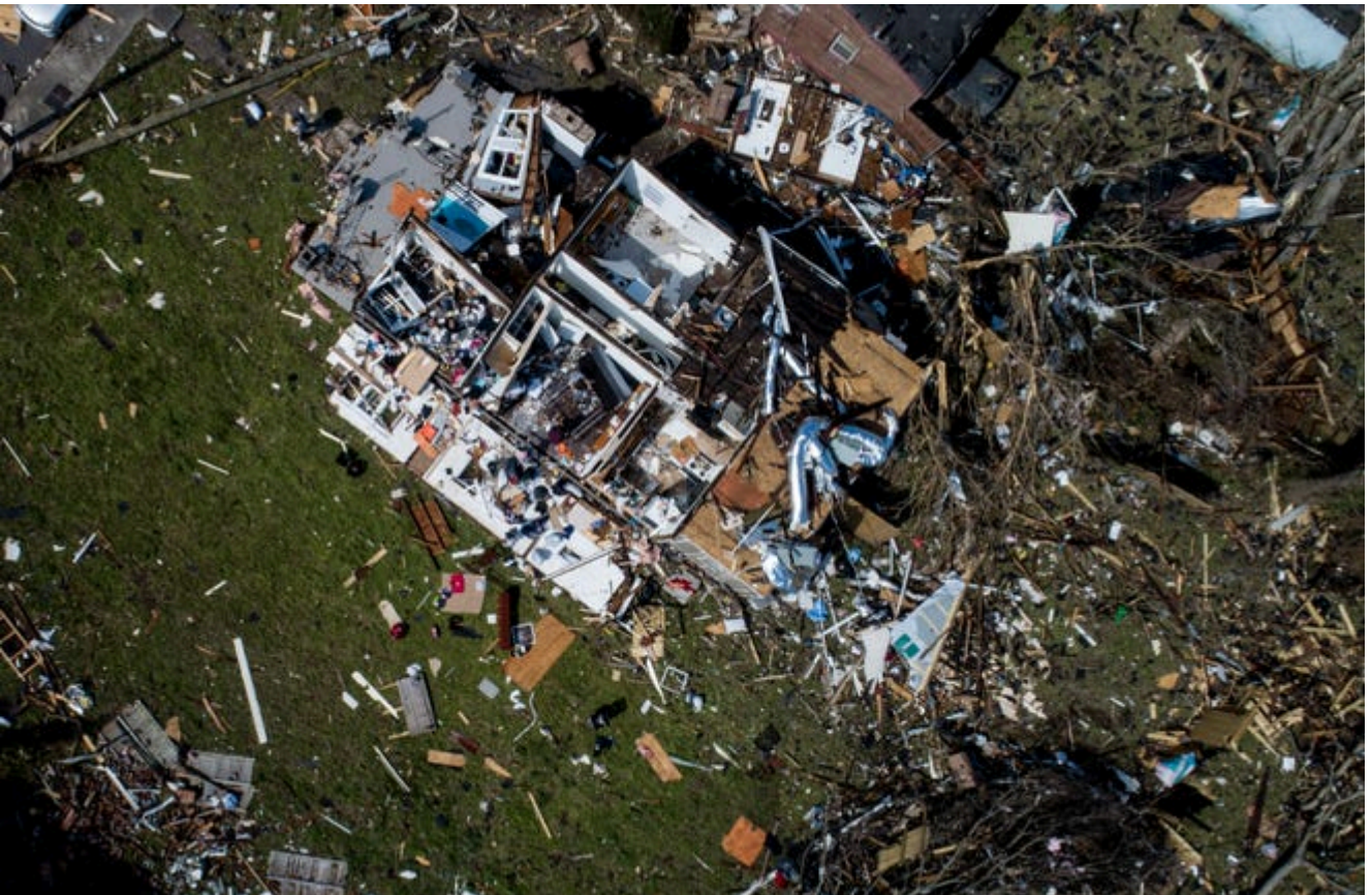
A home was damaged by a tornado in a north Nashville neighborhood. Scott Utterback And Michael Clevenger
