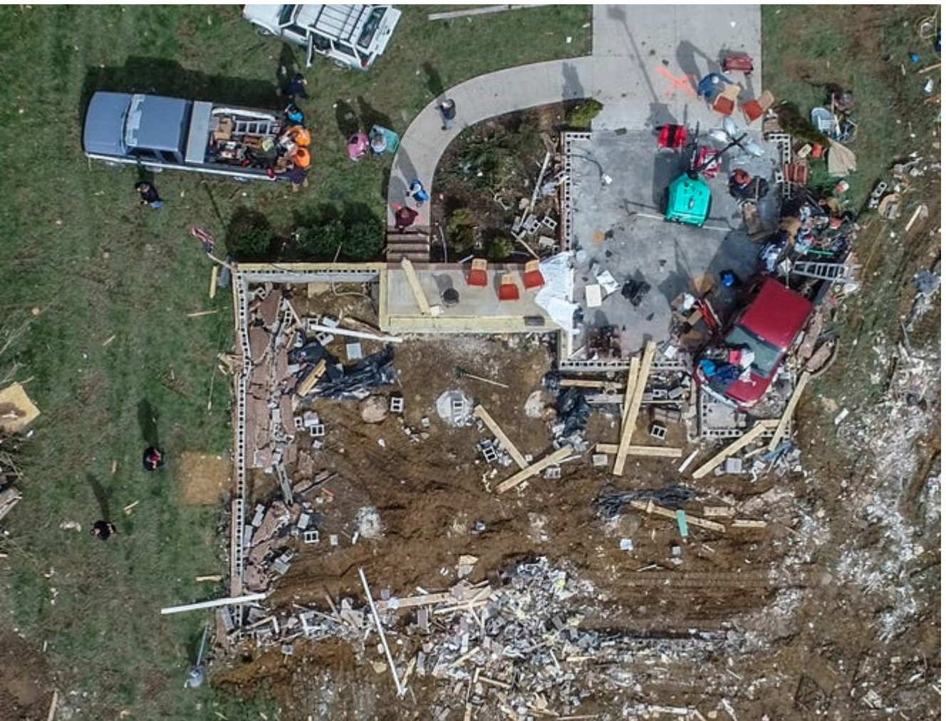
A home near Cookeville, Tenn., was reduced to its foundation by Tuesday's
