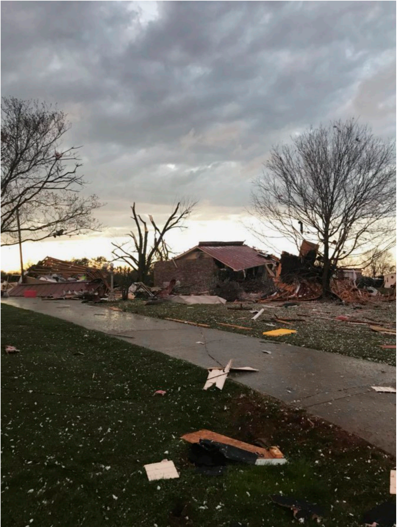
Scattered debris covers the ground in Ardmore, Alabama, on March 19. Severe storms that spawned tornadoes damaged homes and downed trees as they moved across the Southeast on Monday night. Johnny Tribble / via AP On the front end of the system, heavy rain, wind and thunderstorms caused
